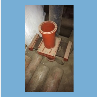
Concrete Saut Of Valve
